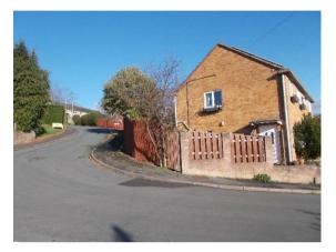
It is three-bedroomed, semi-detached, of brick/concrete construction (including concrete guttering) and would have had wooden doors and windows.
