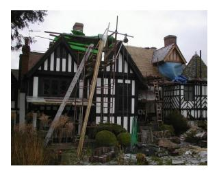
The rotted pine timbers of structurally unsound Victorian additions were replaced by oak framed panels backed with Kingspan and faced with lime mortar.
