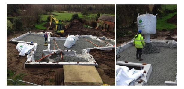
This is commonly used in retrofit buildings. It has good structural ability, drainage, is inert, fire resistant, odourless, no capillary action (prevents soil moisture coming into the building), frost proof and easy to handle.
