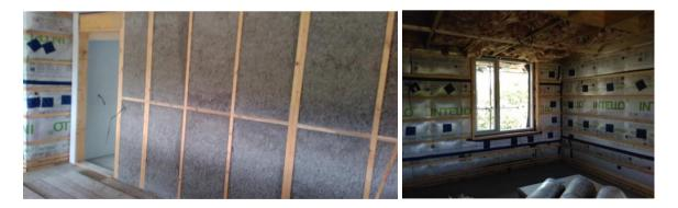
This is a high performance thermal insulation for timber framed houses. The thickness of the insulation is 300mm and it is usually blown into the spaces through holes in the internal vapour control layer. The tight packing of warmcel means there are less gaps for heat to escape in winter or warmth to come in summer. External breathable layers reduce the risk of condensation and mould growth. Our experience is that the structure loses little heat in the winter and keeps cool in the summer.
